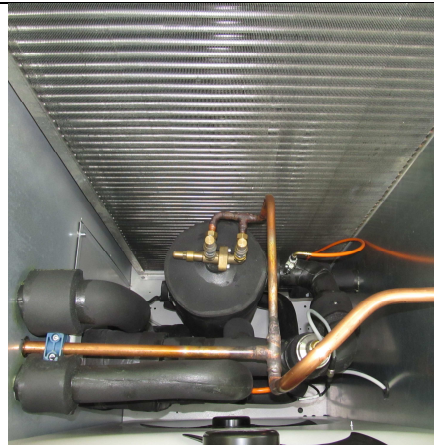
Danfoss high pressure valve arrangement
