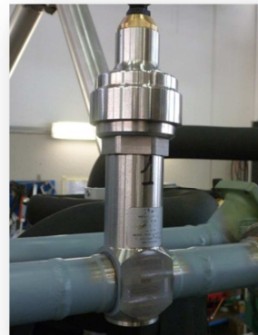
Danfoss high pressure valve arrangement
