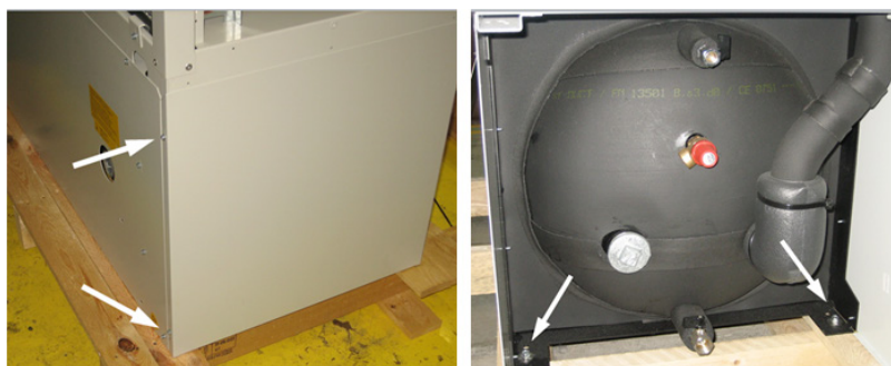
Fig. 8 Details of positions of screws fixing to the pallet for units with tank
