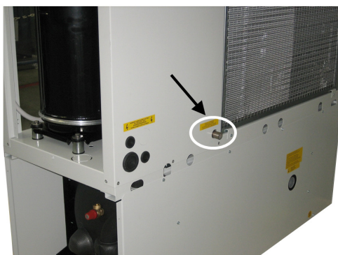
Fig. 1 Position of condensate drain
